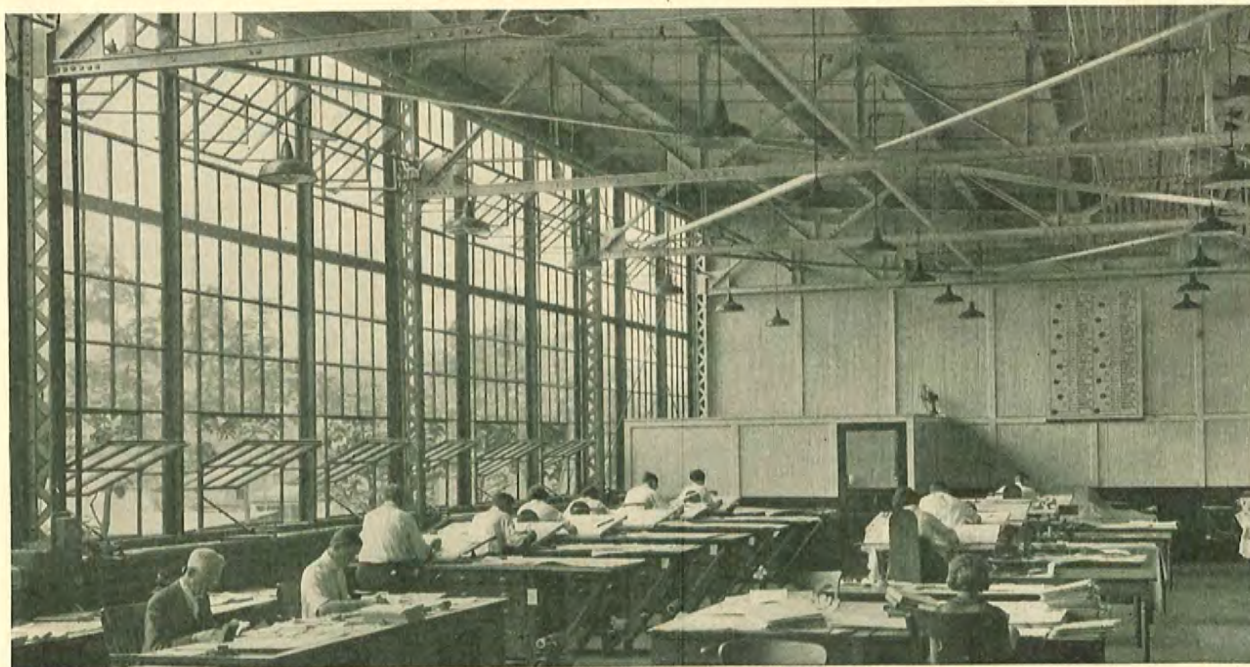
Lupton Operating Device, controlled by hand chains, is used to operate the upper ventilators of Lupton Pivoted Windows in this drafting room.
