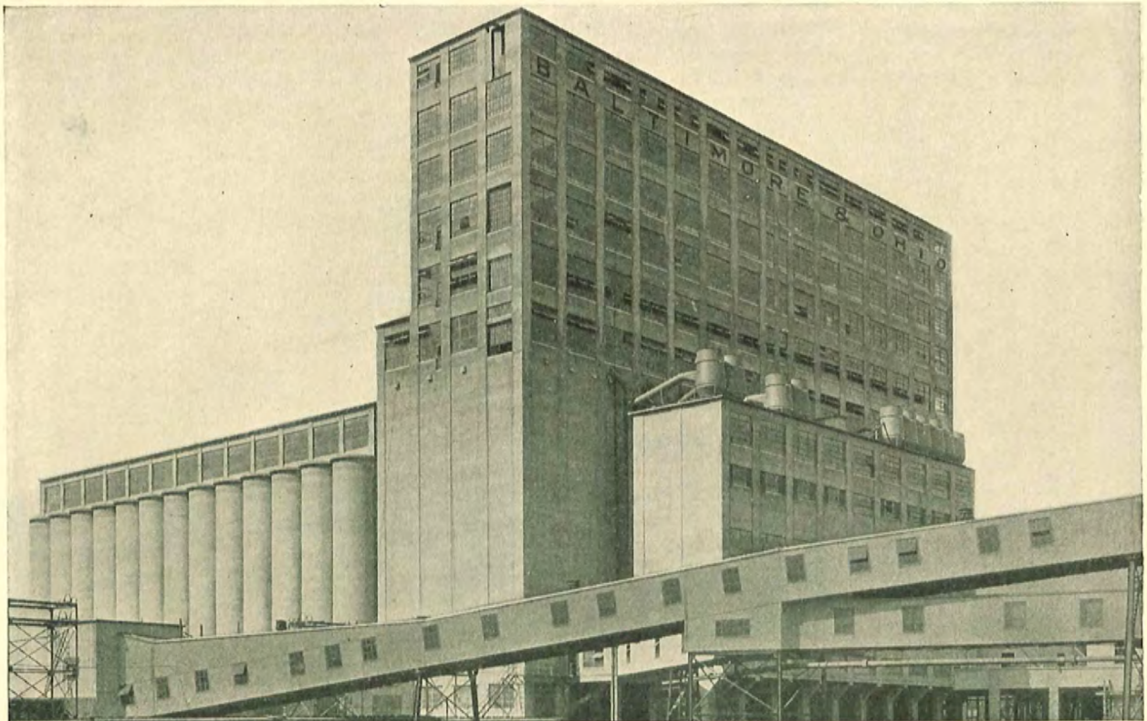
Baltimore & Ohio R. R. Grain Elevator Baltimore, Md.
