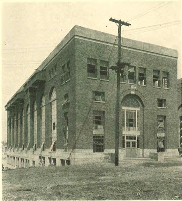
Lupton circle head Pivoted Window units, used in the Acme Power House, Toledo, Ohio
